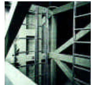
Interior Section of a Tower
